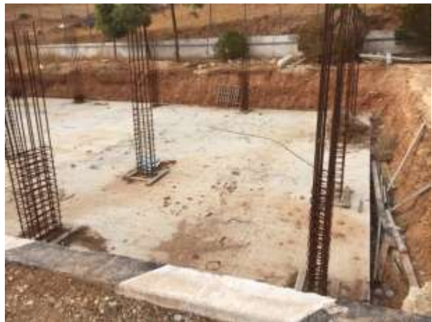
Foundation for the school in Furush Beit Dajan
